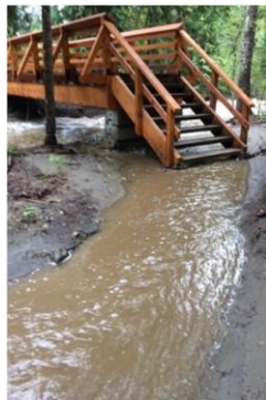
Mill Creek Regional Park AFTER 2017 flood
