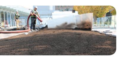
Manually placing soil can be a time consuming task, and if not performed properly can damage the surrounding environment. We provide professional installation services using our blower trucks with skilled, experienced experts. This ensures the soil is spread evenly, there is no damage to lawn areas and best of all, it saves you time to work on other projects or relax!
